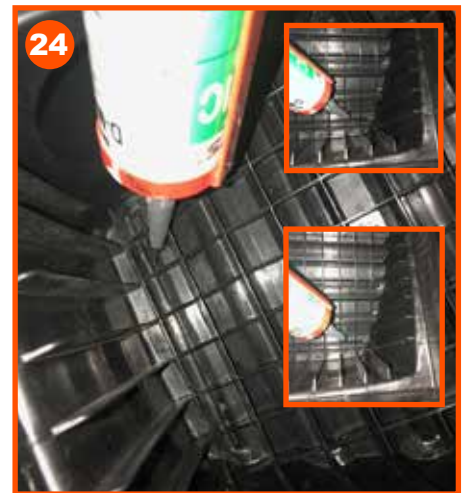
24 Seal any holes inside the air box with Butal mastic sealant.
