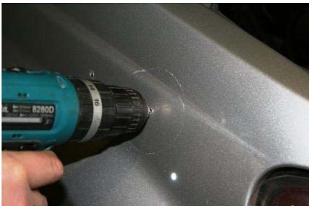
3.38 When pre-drilling the snorkel hole, ensure that the hole goes through the inside panel as well.
