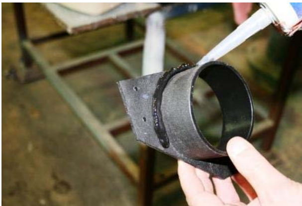
3.24 Remove the SP210 and apply some mastic as shown
