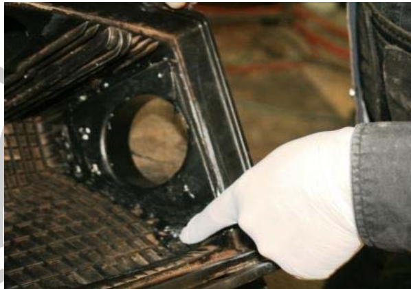
3.24 Remove the excess mastic for a smooth finish
