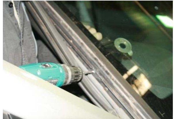
3.58 Using a 4mm bit, pre-drill the two holes
